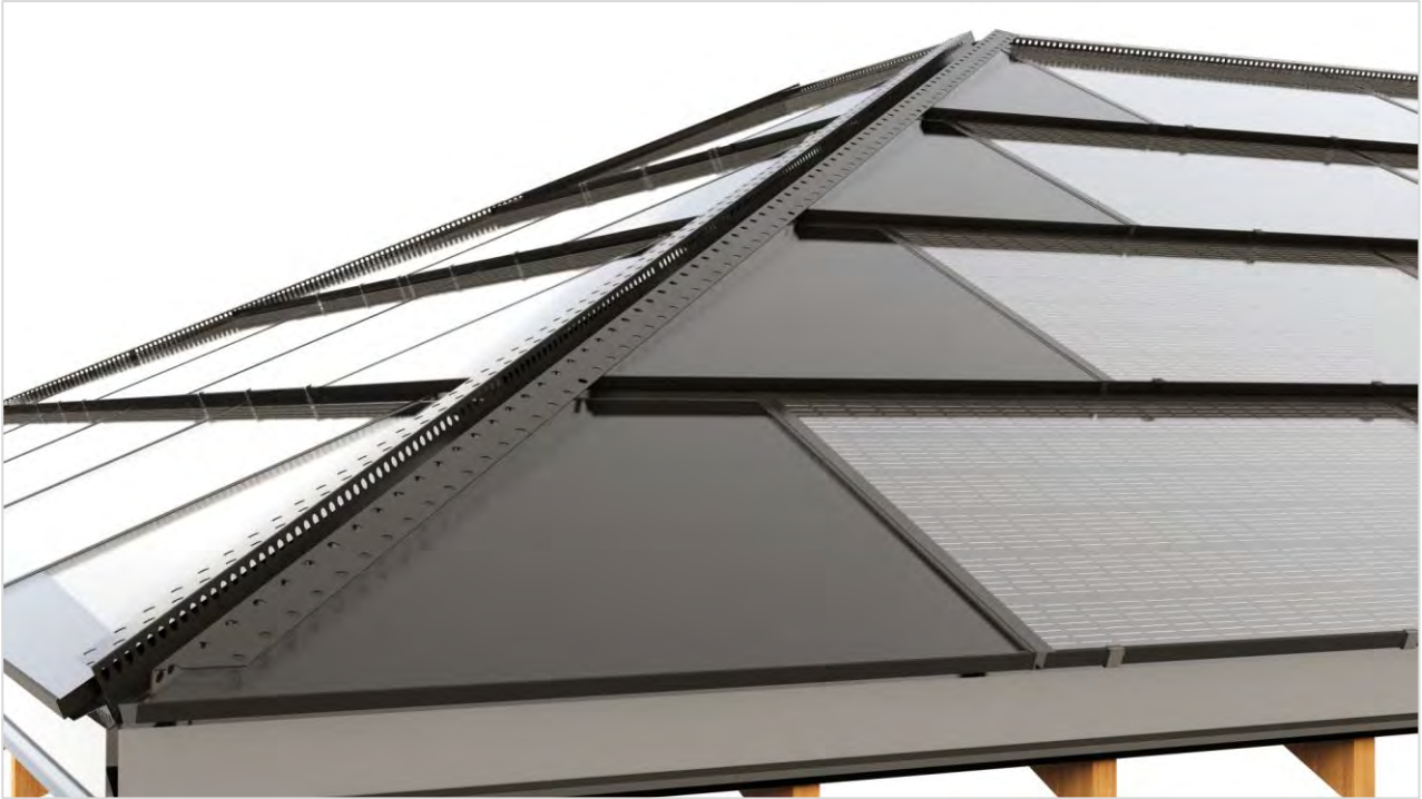
Continue installing FILLER-panel (dummy) panels up to the ridge.
