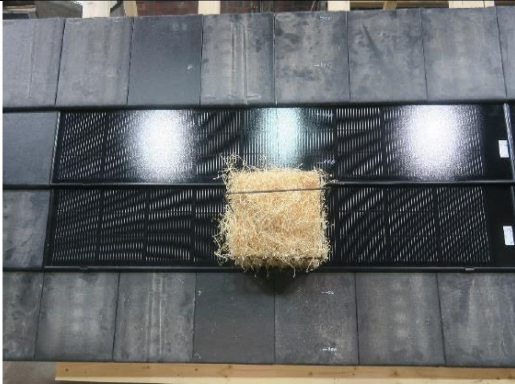
Fig. 21: Solarstone tiled roof kit, Test set-up (test 2)
