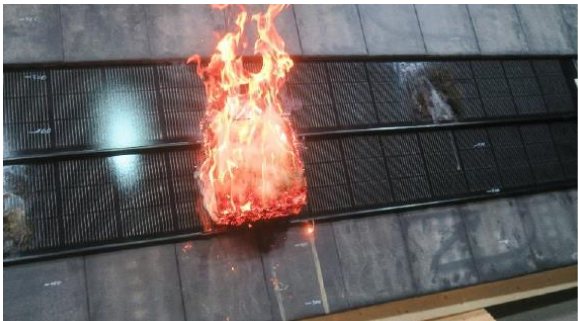
Fig. 26: Solarstone tiled roof kit, Test set-up (test 3) - Ignition
